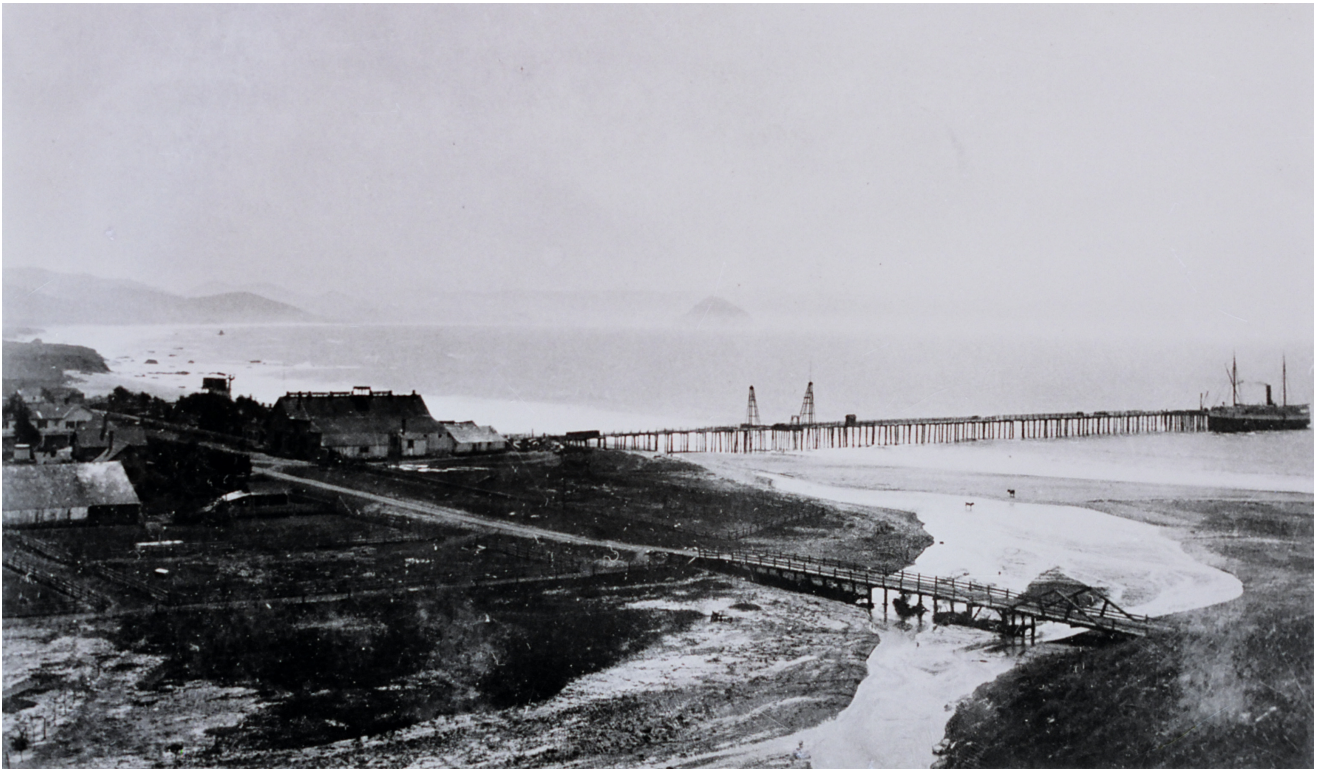
View to southeast showing 1878 wooden bridge over Cayucos Creek, Cass Landing and pier, circa 1878-1890. (Courtesy of the Friends of the Cayucos Library—Sam Borradori Collection).
